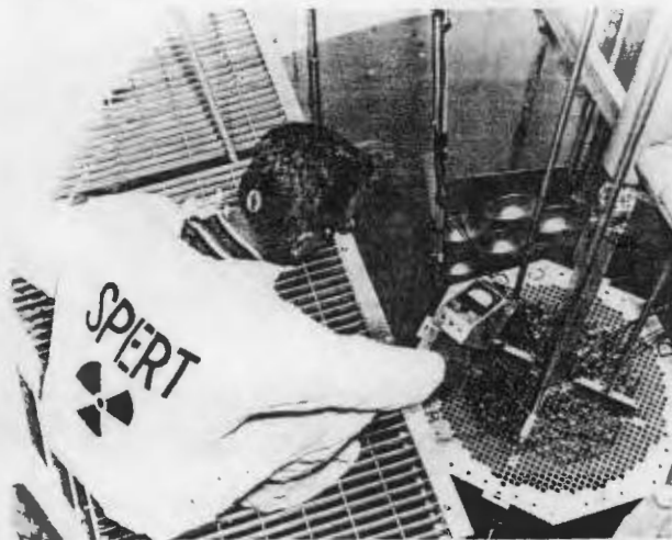
SPERT-I URANIUM OXIDE FUEL CORE
