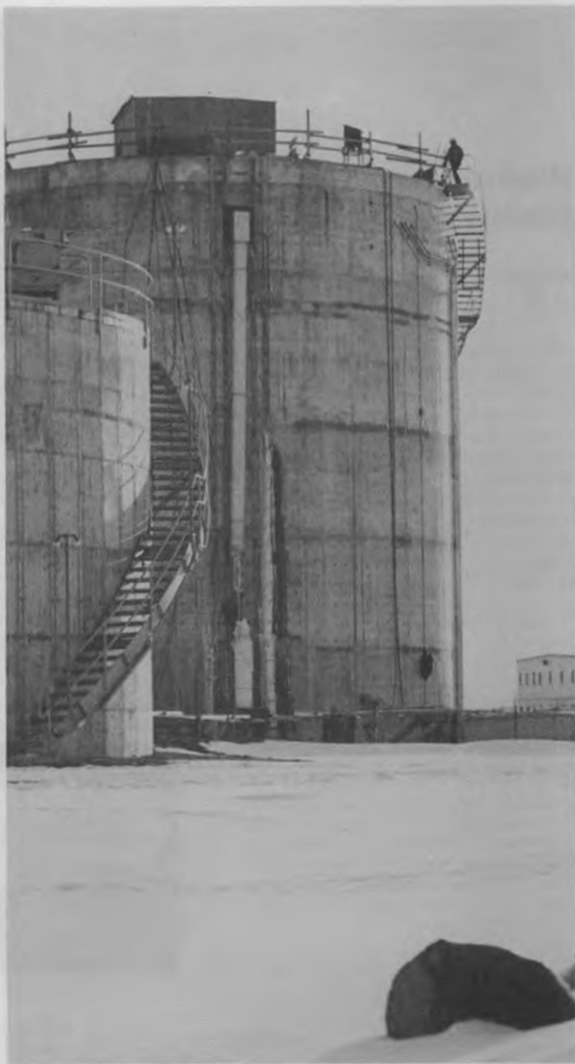
Two bin sets for storing calcined high-level radioactive waste at the ICPP. The plant celebrated 25 years of calcining in 1988.
