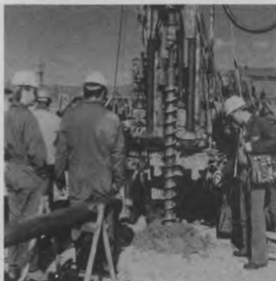
Sampling of the Test Support Facility injection well.
