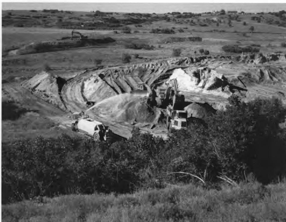
Uranium mill tailings at Monticello, Utah, are excavated for disposal offsite.
