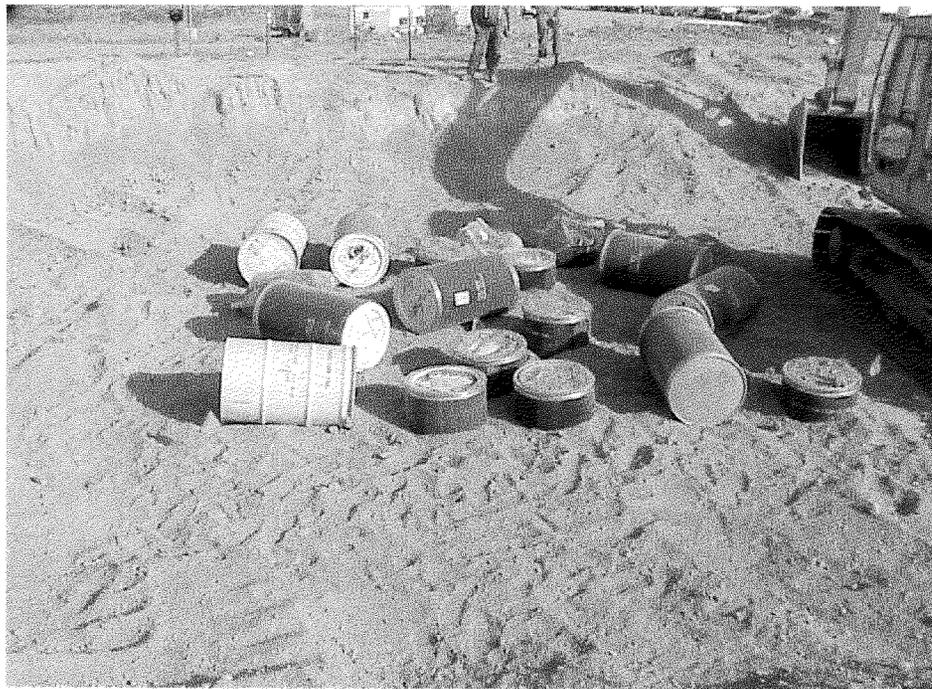
Figure 49. Top layer of in situ grouting pit during construction with white nitrate drum in corner.
