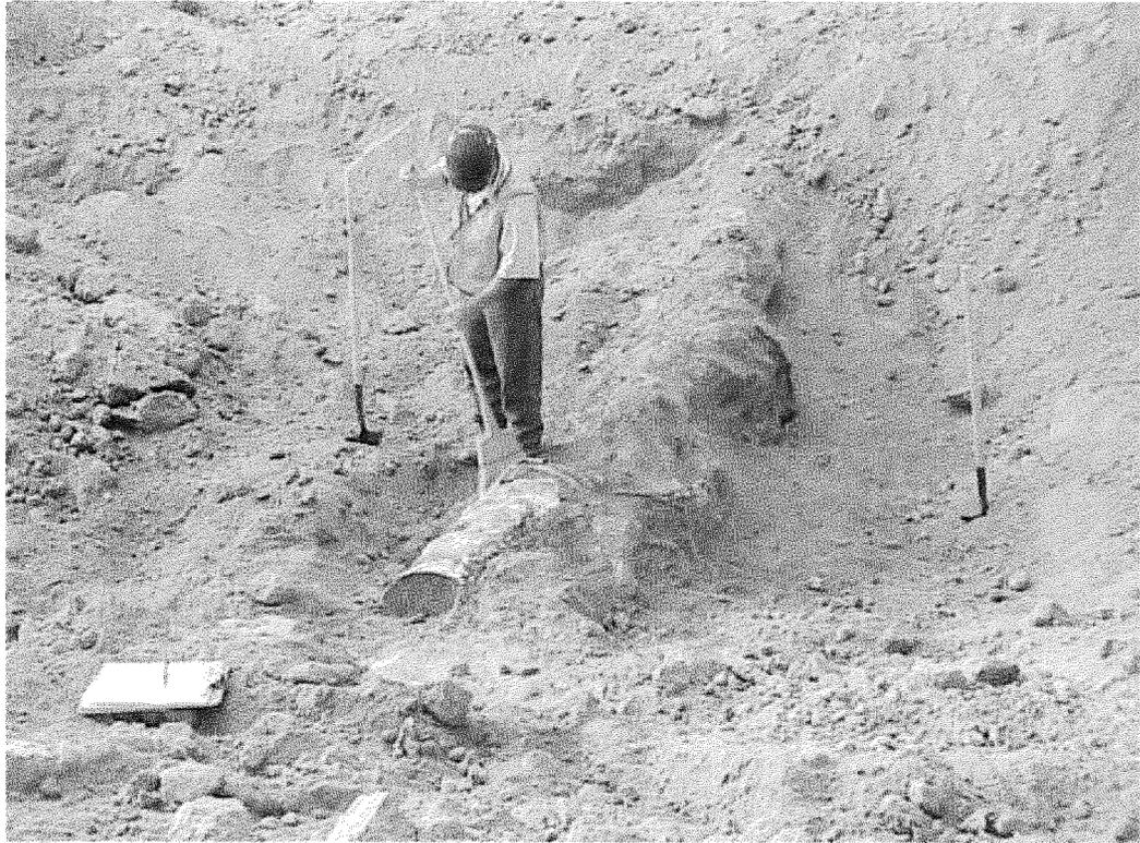
Figure 48. Top of monolith showing grouted drum embedded in northwest edge.
