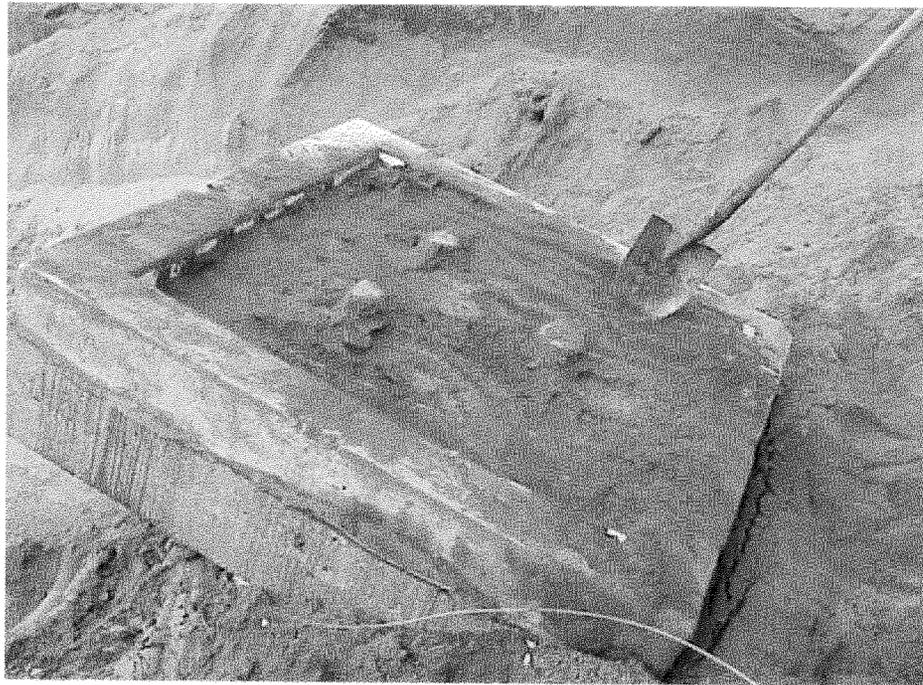
Figure 23. Underside of U.S. Grout thrust block.
