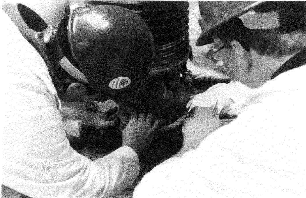
Figure 44. Placing plastic sleeve material on drill string stinger (Photo PN01-520-4-10).
