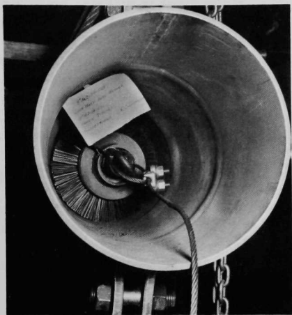
Figure 6. Ten-inch Cleaning Plug in Header
