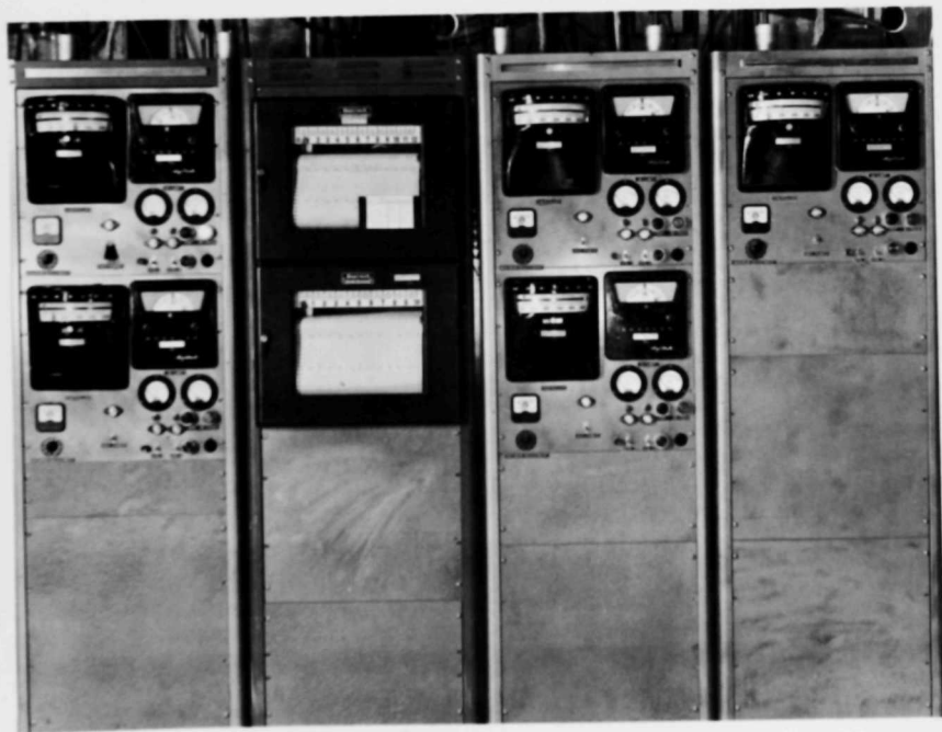
Figure 9. Controllers and Recorders Installed in the Basement of the CP-5 Reactor for Operation of Irradiation Experiments in Five Vertical Thimbles.
