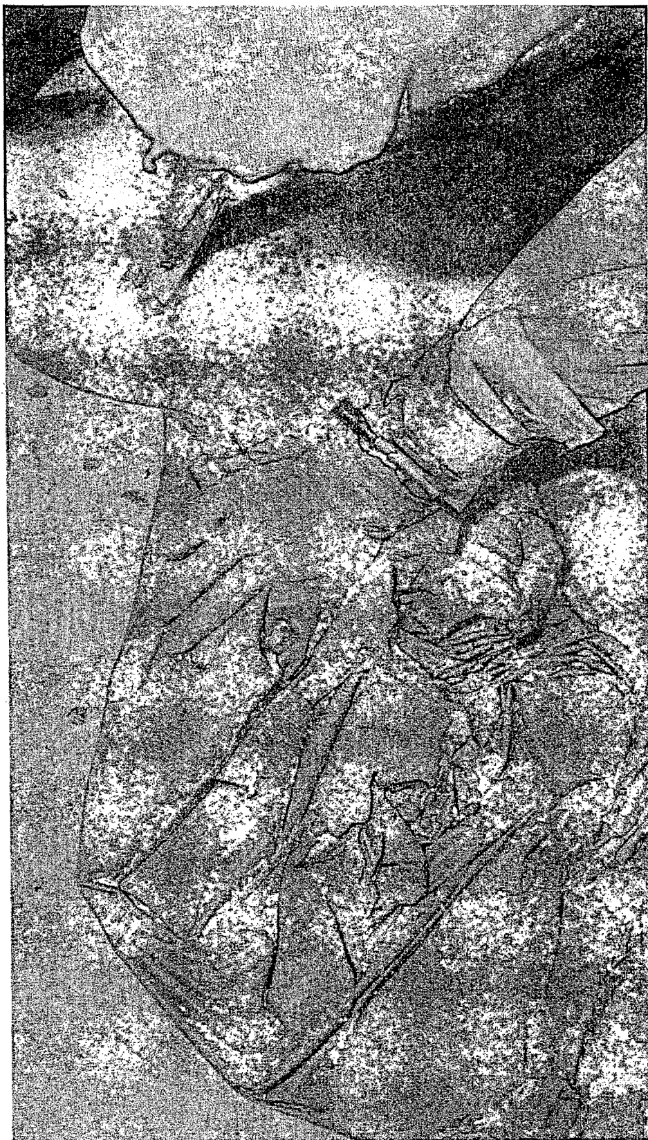
Figure 8 Technician removes strippable coating from Reactor Building floor.
