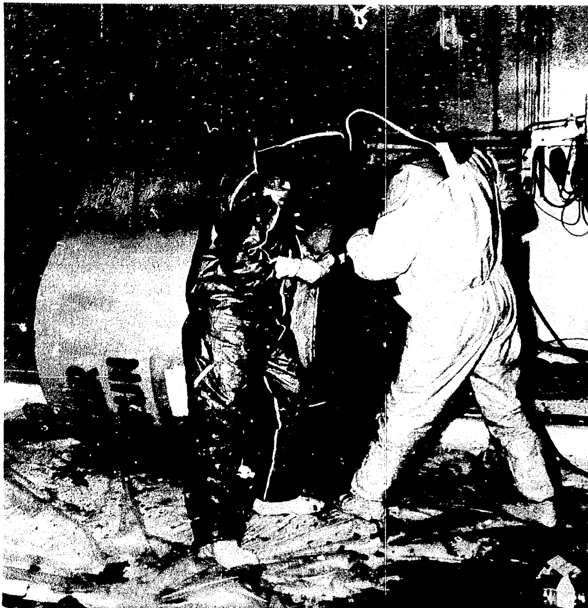
Figure 5. Removal of a study section from liner PF-16 using a portable reciprocating saw.
