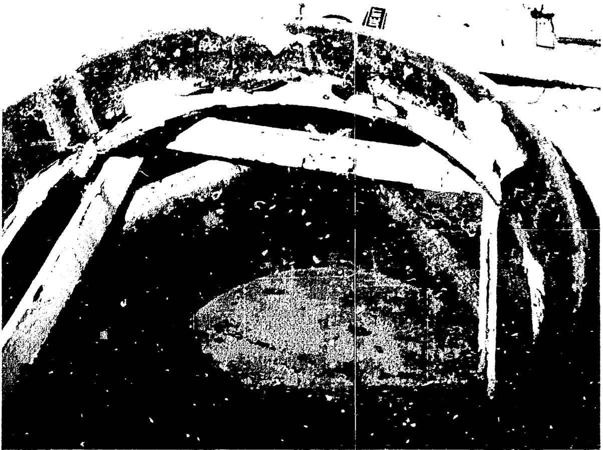
Figure 9. View of manway port of liner PF-16 showing extensive coating damage.
