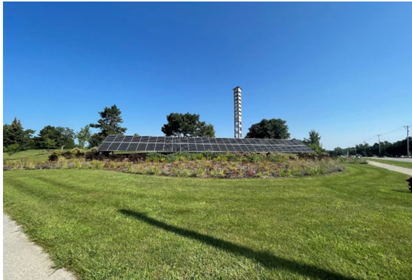
Figure A-1. A behind-the-meter ground-mount solar system at a municipal building in Meridian Charter Township, Michigan. (Photo by Sharlissa Moore.).
