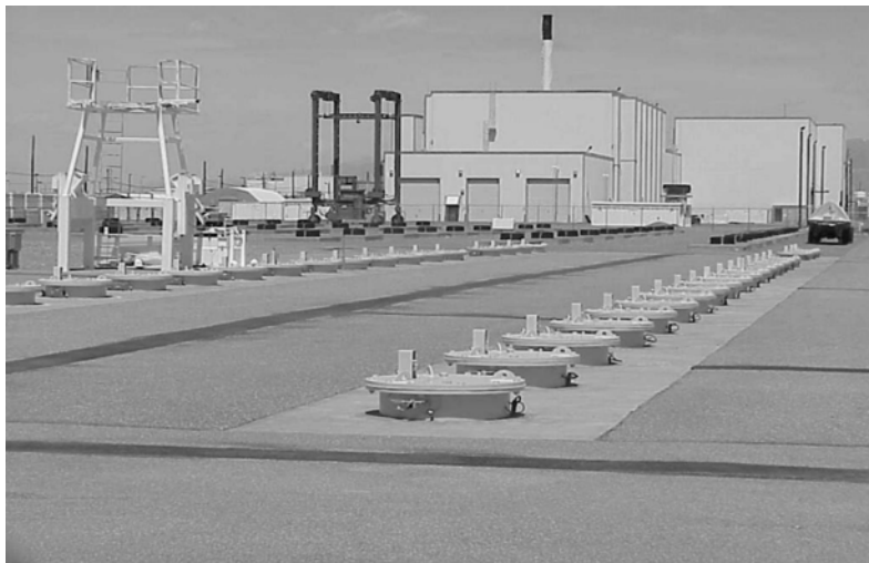
Figure 3. The Below-grade Storage Facility CP-749 at the INL Used to Dry Store Peachbottom Reactor SNF
