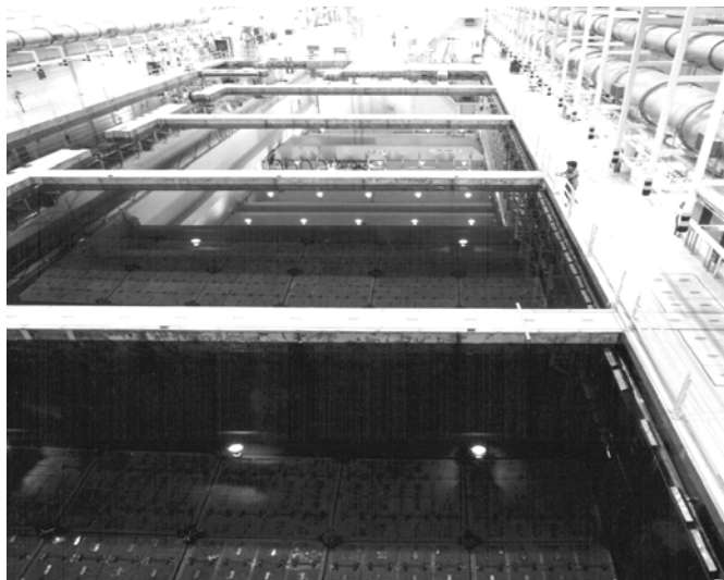
Figure 1. The modern steel-lined CP-666 Storage Pool at the Idaho Nuclear Technology and Engineering Center (INTEC)
