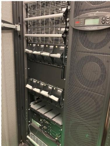
Figure 5: The eight UPS batteries used for peak shaving.
