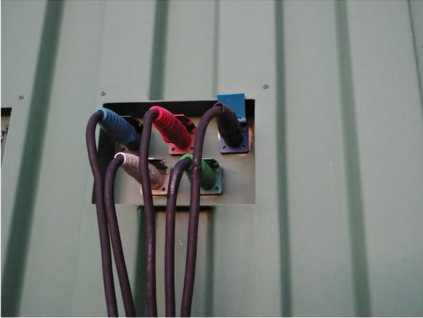
**Figure 3: The datacenter is 208 volt three-phase and single panel fed for all HPC systems and cooling.**
