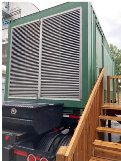
**Figure 2: Self-contained datacenter hosting the three classes of HPC hardware, stand-alone cooling system, and UPS battery backup.**
