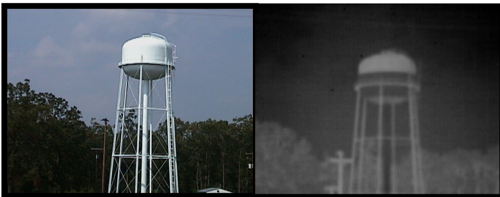
Figure 3-2. Visible Image, on left, of Water Tower During Summer Morning and Infrared Image, on Right, Taken at Approximately the Same Time Showing the Tank’s Liquid Level
