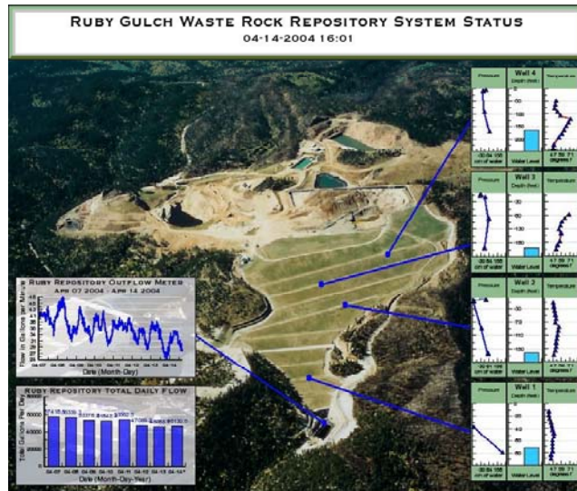
Figure 5. Example of the real time data observations at the Gilt Edge mine site.
