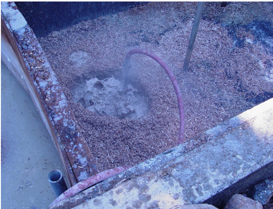
Figure 3. Injecting Compressed Air in the Apatite II TM Media.
