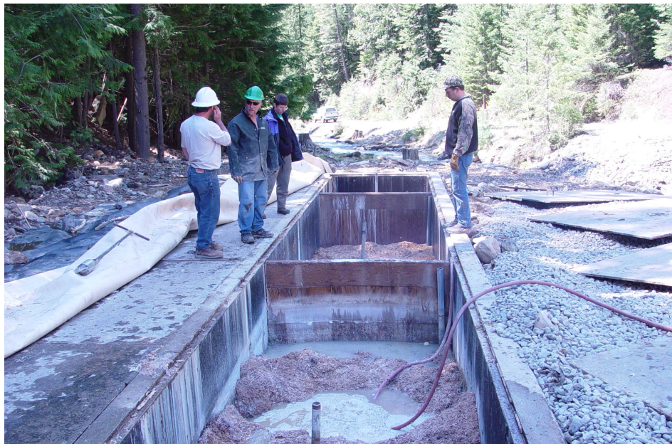
Figure 2.0. Construction of the Reactive Barriers at the Success Mine Site.
