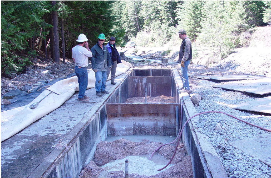
Figure 10. Injection of Compressed Air into the Reactive Media.
