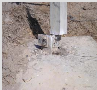
Figure 1: Images from recent transmission tower attacks. The image on the left is from news reporting on two towers that were downed in Oak Creek Wisconsin on October 9, 2004. These towers collapsed after having the bolts removed at the base of the towers. More extensive damage occurred to distribution networks in Iraq (images on right) when towers were toppled and destroyed to get at the transmission cables for the recyclable metals.
