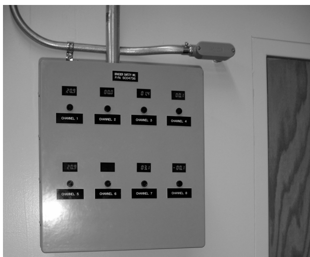
Fig. 3. The auxiliary readout panel in the lab office area.
