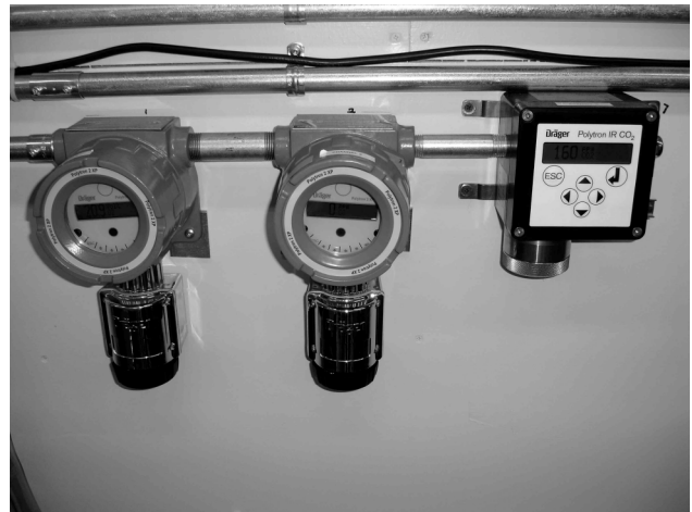
Fig. 4. O 2 , CO, and CO 2 sensors used in the NHI lab. The sensors are located on a wall near each experiment area.
