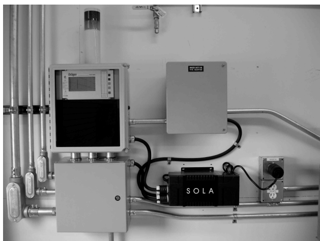
Fig. 1. The NHI lab hazardous gas system controller.
