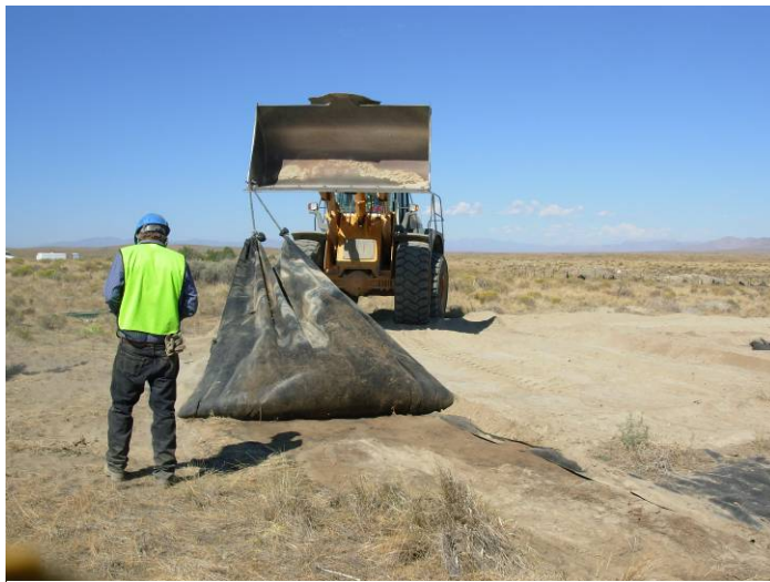
Figure 29. Geotextile fabric is removed from the surface of 10-BT-2189 at the BLR-8 trench area.
