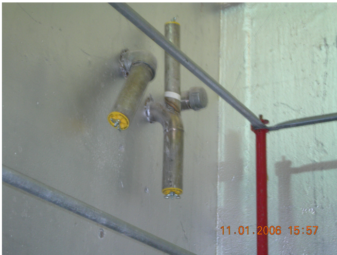
Photo 5 Plugged Pipes
