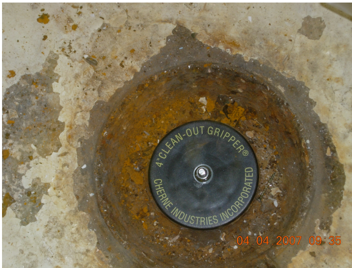
Photo 4 Plugged Floor Drain
