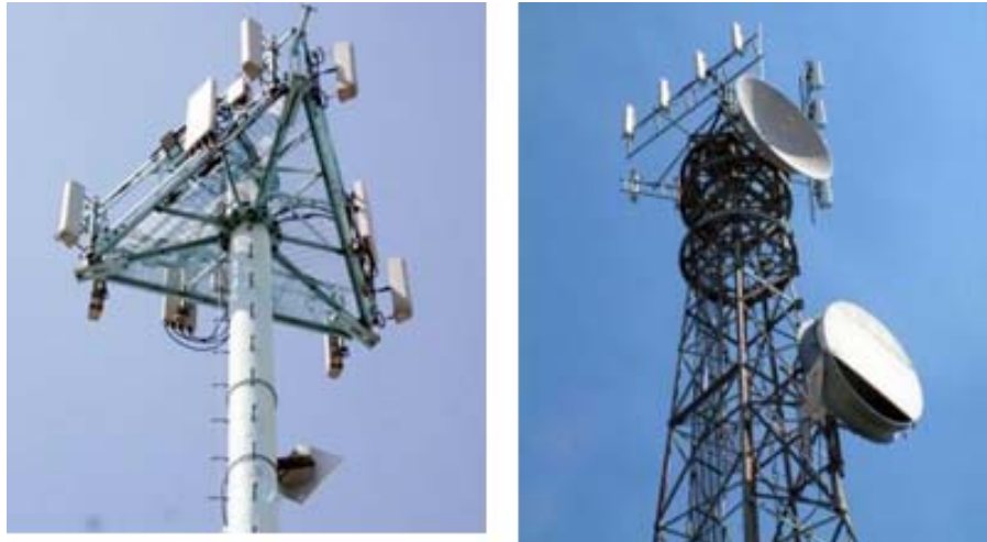
Figure 2-8: BTS Antennas and Microwave Backhaul
