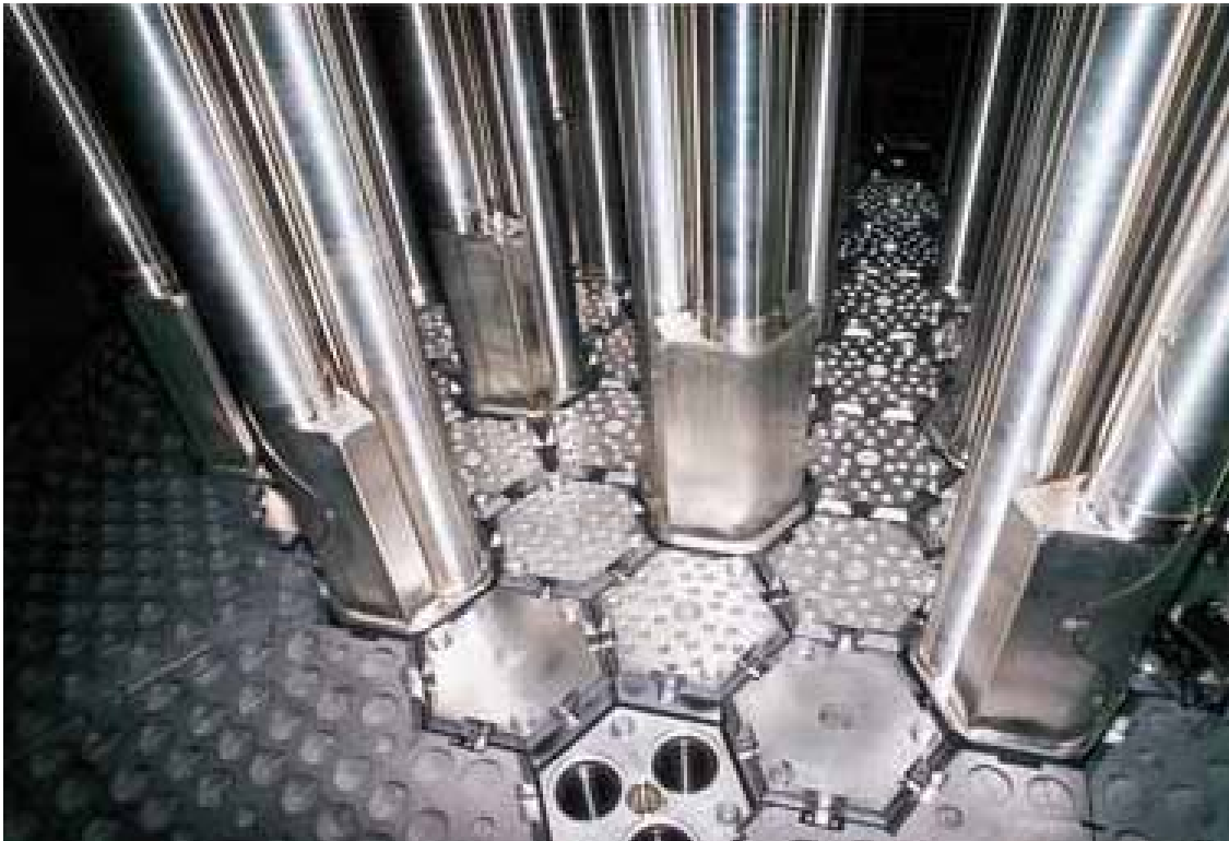
Figure 1.70. Inside of the Reactor Pressure Vessel. a
