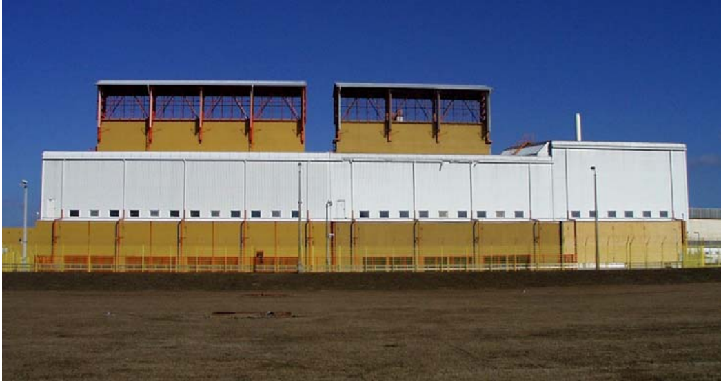
Figure A-6. Paks MVDS in 2000 showing natural convection cooling exhaust outlets (Ordogh et al. 2004).
