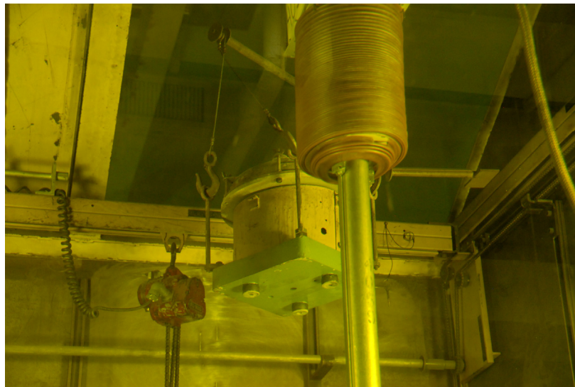
Fig 3. Removing existing polisher through 'containment-box' roof
