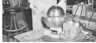
Reconstruction of 1946 criticality accident with beryllium reflectors
