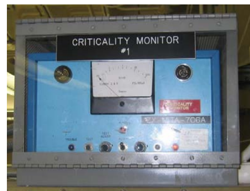
A criticality alarm system monitor at MFC. Criticality alarm activation signals a need for immediate evacuation.
