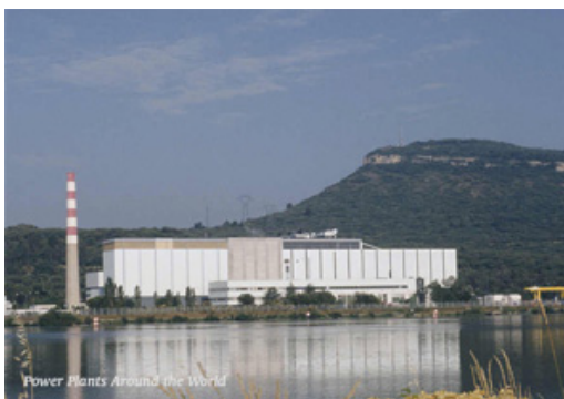
Figure 2-7. The sodium-cooled fast reactor Phenix has served French research and development programs for decades. The Department of Energy currently has advanced fuel experiments under irradiation in Phenix.
