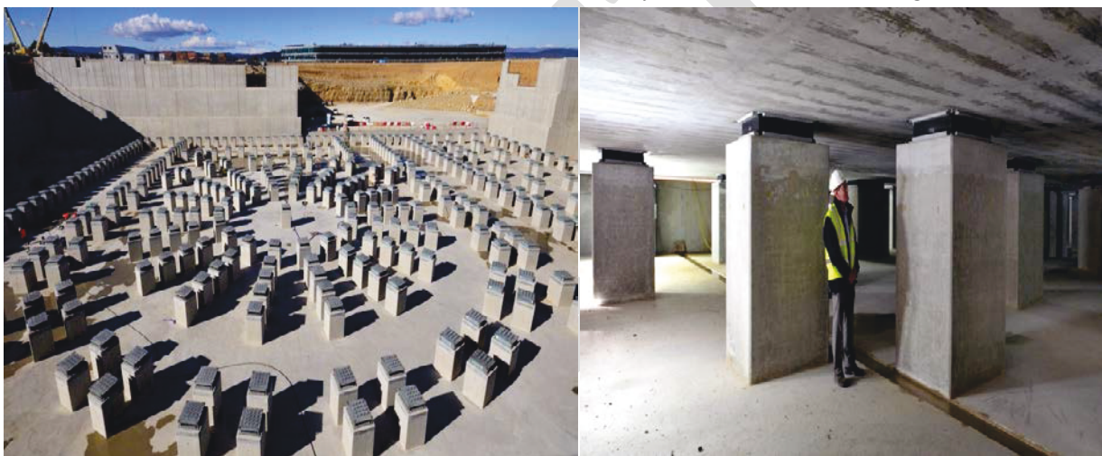
Figure 3 Seismic Isolation for ITER and JHR
