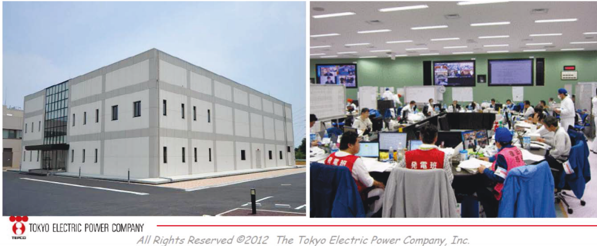
Figure 2.3.10: Seismically isolated emergency response building placed at the Fukushima Daiichi site
