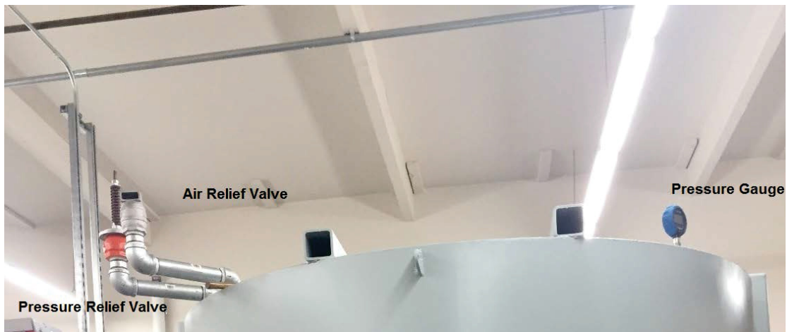
Figure 5. PET reliefs and pressure gauge.
