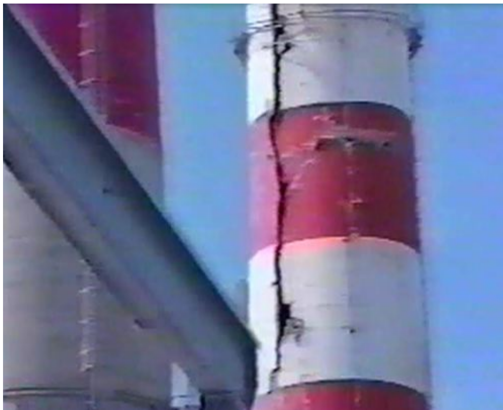
Figure 1. Structural damage to Turkey Point Unit 1 exhaust stack. (Union of Concerned Scientists 2011).
