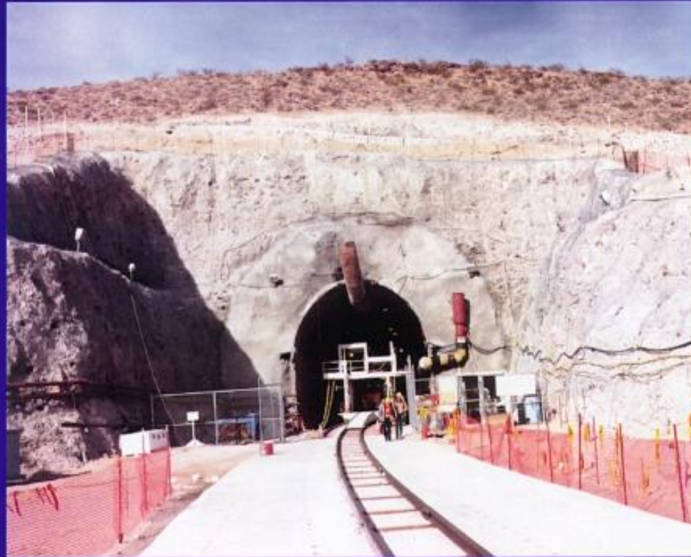
STARTER TUNNEL ENTRANCE AT YUCCA MOUNTAIN
