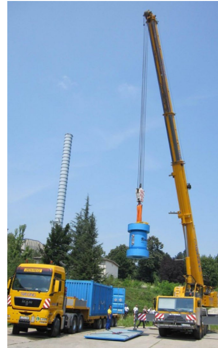
VPVR/M cask placing into an ISO 20ft container
