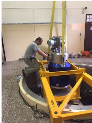
Installation of the transfer cask above the MNSR pool
