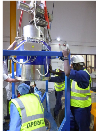
Transfer cask installation
