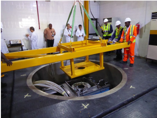
Equipment installation over the reactor pool
