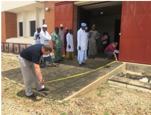
Outer and inner gates ramp without a horizontal platform near the gate
