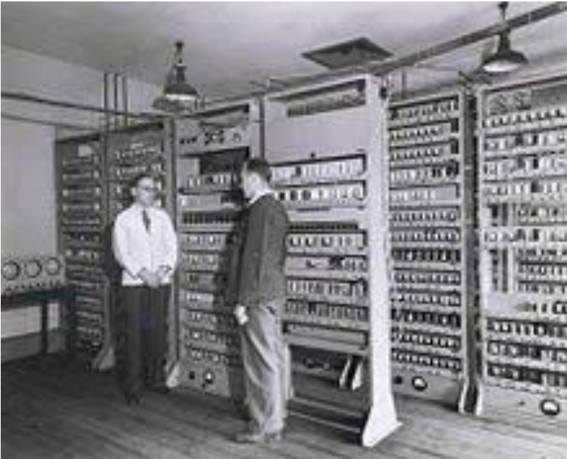
The Electronic Delayed Storage Automatic Calculator (1949). Peak performance: 600 instructions/sec
