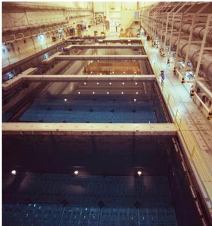
Figure 18: Five of the six interconnected CPP-666 storage basins.
