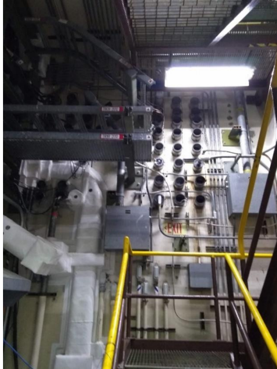
Figure 5-8 More Penetrations in the Reactor Building ( Courtesy of Oyster Creek NPP )
