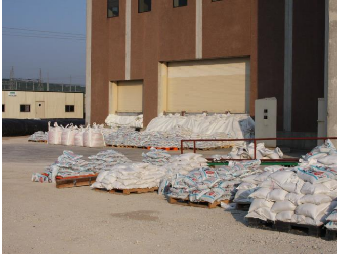
Figure 4-11 Sand Barrier Used in Fort Calhoun Station During the 2011 Flood Event [43]
