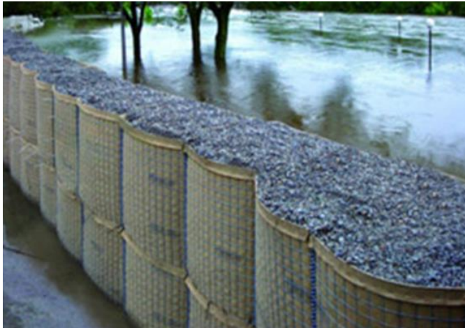
Figure 4-11 Sand Barrier Used in Fort Calhoun Station During the 2011 Flood Event [43]
