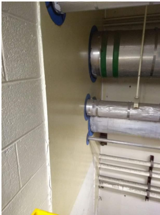
Figure 5-7 Penetrations in the Reactor Building (Courtesy of Oyster Creek NPP)
