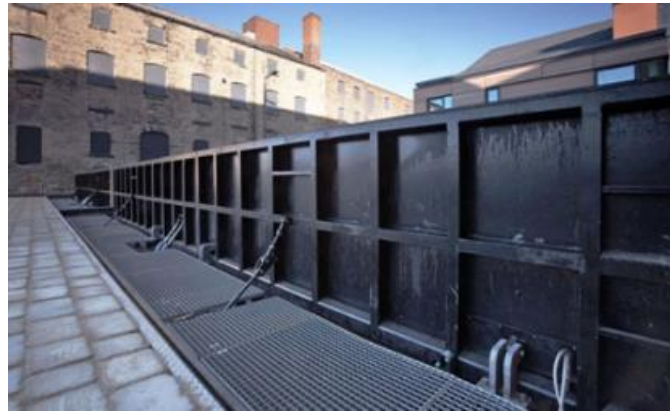
Figure A-4 Hydraulically Activated Barrier [70]
