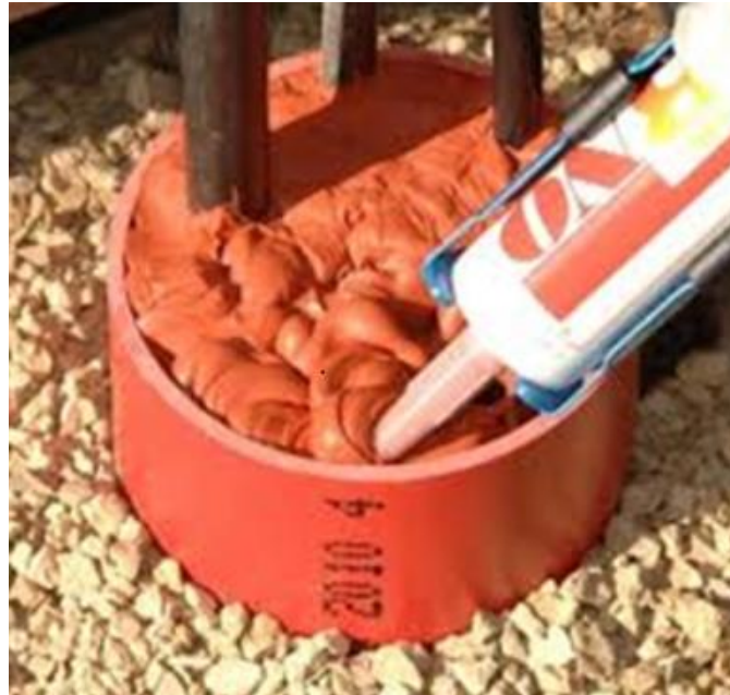
Figure 4-2 Vulcanizing Foam Seal [38]
