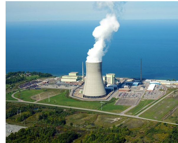
Nine Mile Point (Courtesy of Exelon)
