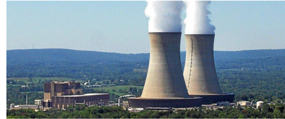
Limerick Generating Station
