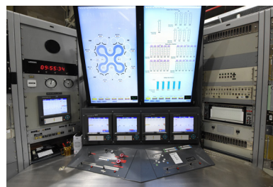
ATR's control console was replaced in FY20, improving reliability in support of reactor operations.
