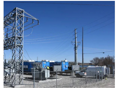
In March 2021, INL led a team and worked with Idaho Falls Power, the municipal utility serving Idaho Falls, to demonstrate the ability to blackstart five run-of-river hydropower plants and serve critical loads (like hospitals, fire stations, emergency shelters) when the transmission system is experiencing an outage.
