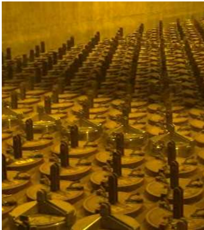
Figure 2. The tops of fuel storage canisters inside the CPP-603 fuel storage area rack
