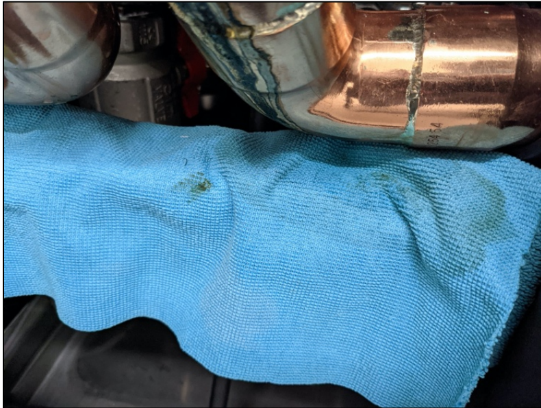
Figure 3. Leak of cooling water in CDU 1. Picture taken November 8, 2021.
