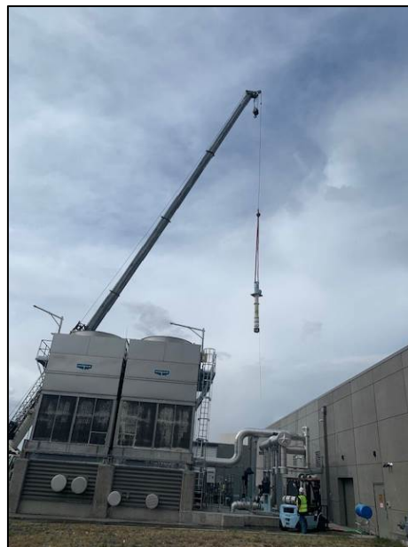
Figure 2. Pump 8 was removed for repair on October 18, 2021, leaving only one operational pump in the cooling tower water basin.
