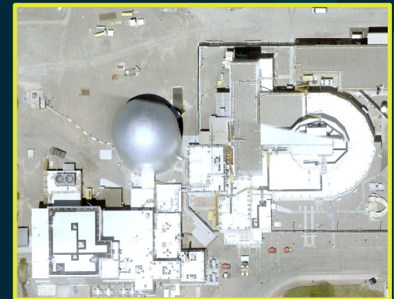
Location of the DOME at INL's Materials and Fuels Complex
