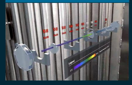
Overlaying predicted temperature values from a machine learning algorithm on a digital representation of a real asset using mixed reality
