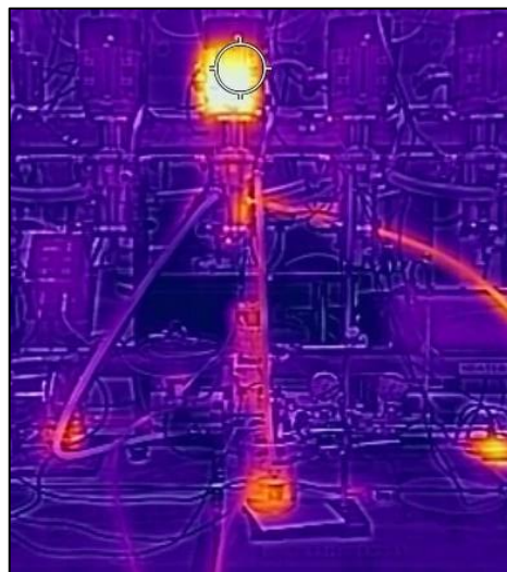
Figure 2. Infrared thermal image of single contactor operation.
