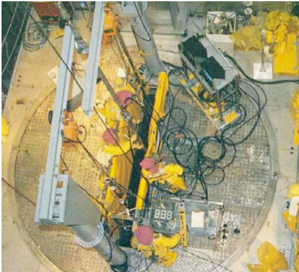
Figure 49. Photos of shielded defueling work platform. (Courtesy of NRC/INL tmi2kml)
