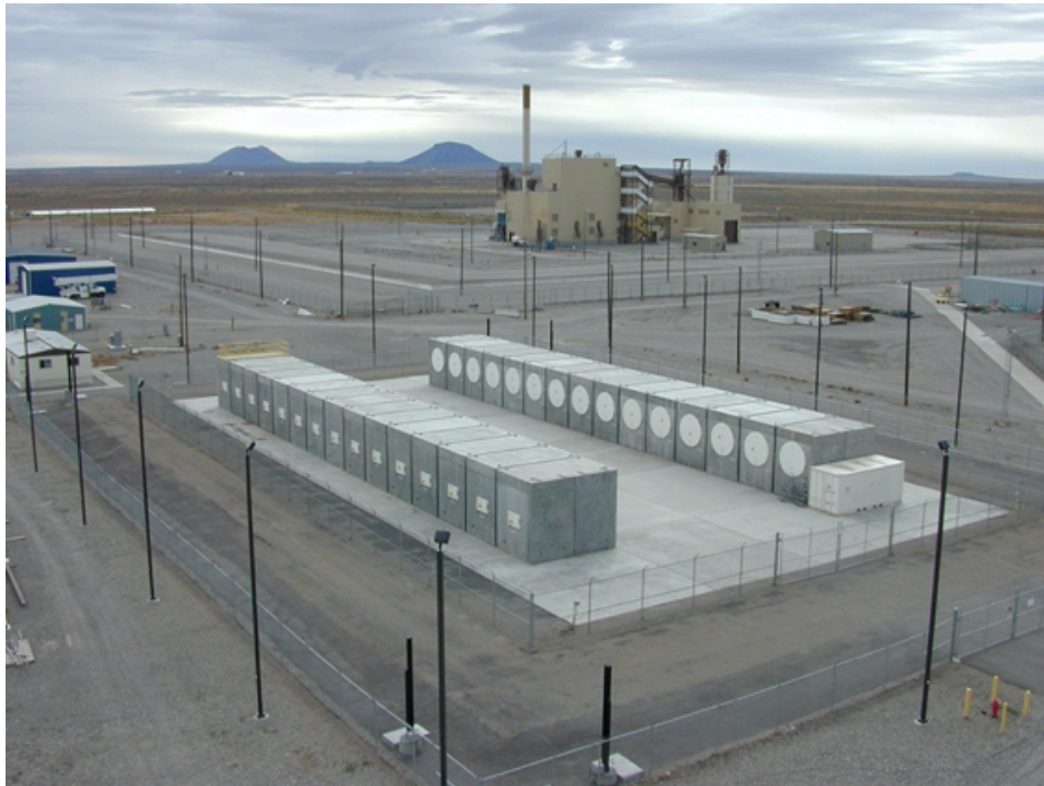
Figure 100. CPP-1774 ISFSI with HSMs. (Courtesy of INL)
