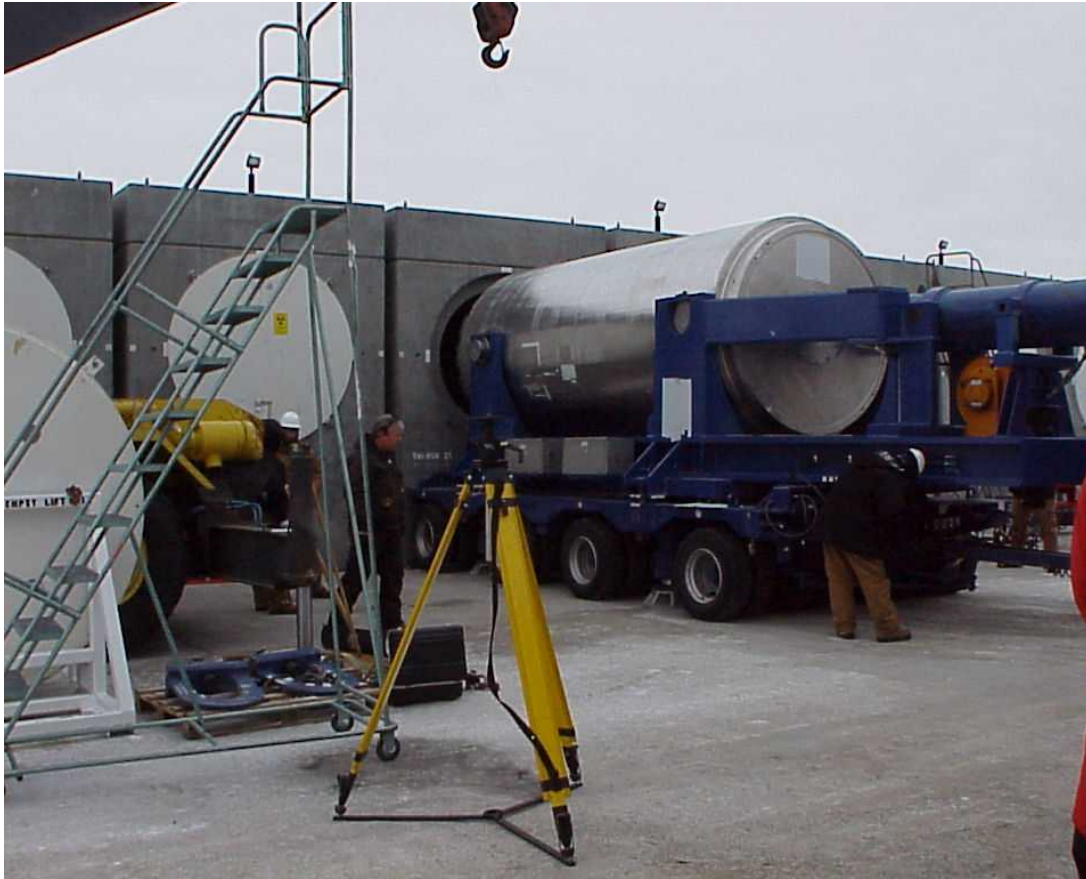
Figure 98. Mating OS-197 to HSM at INTEC CPP-1774 ISFSI for DSC placement. (Courtesy of INL)
