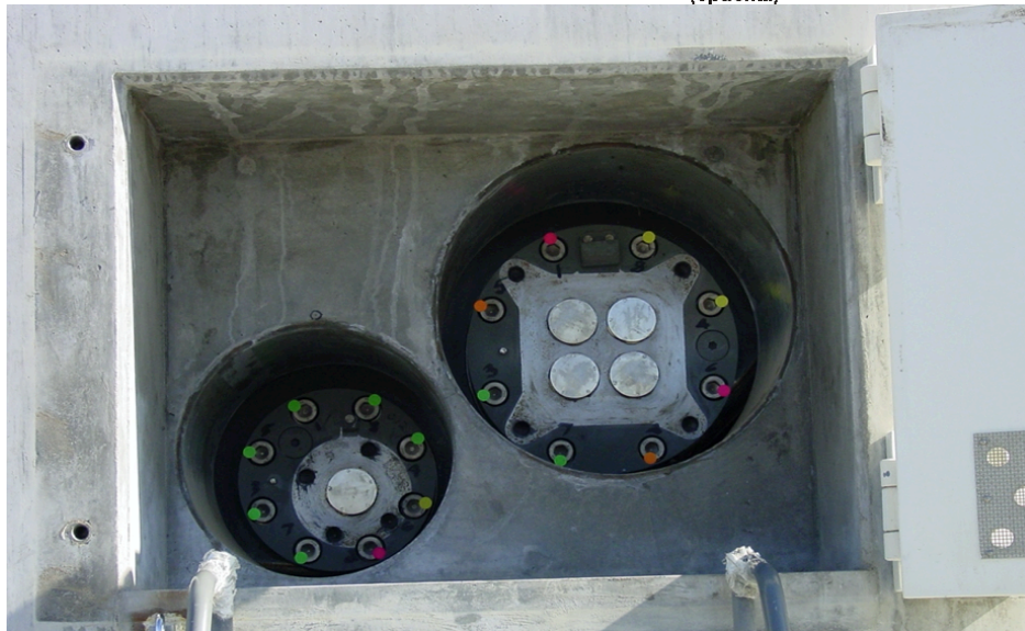
Figure 99. HSM cutaway diagram (top) and photograph showing purge vent and filter port (bottom). (Courtesy of INL 2002).
