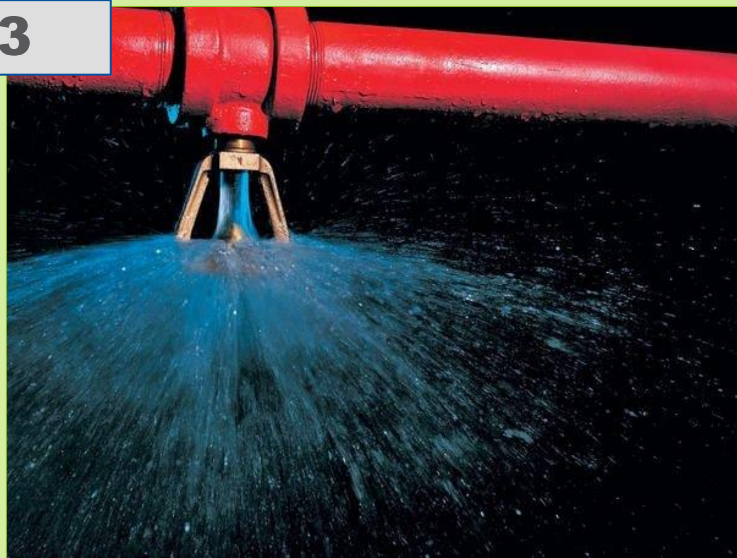
Typical fire sprinkler Eduardo Villafuerte, Why Fire Sprinklers Fail, 2019
