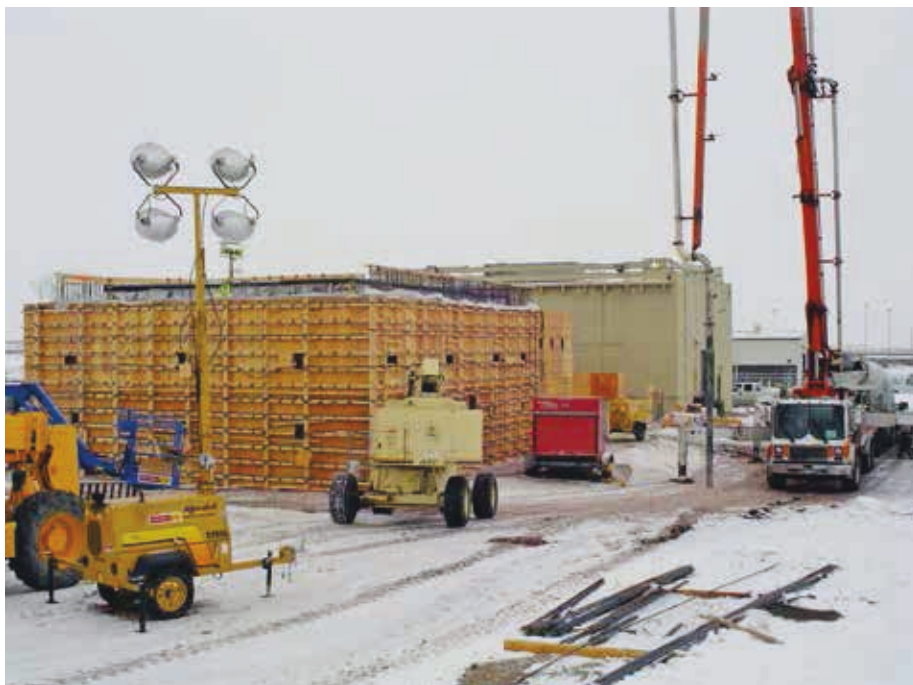
Equipment set up to pour concrete for the walls of the new SSPSF. (Photo: INL RPS Program)
