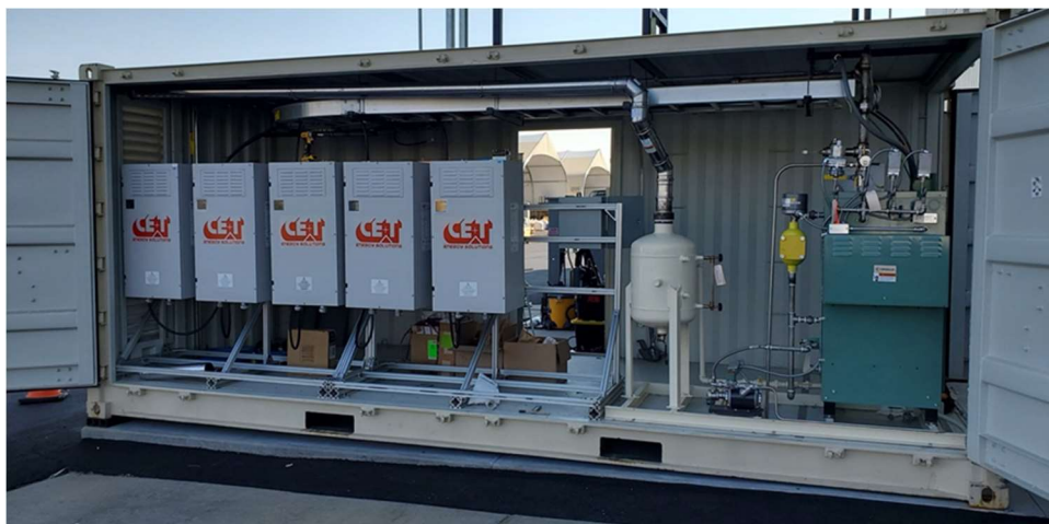
Figure F-1. INL’s High Temperature Electrolysis (HTE) Support Facility with doors open showing the CE+T power converters and the Chromalox steam generator.
