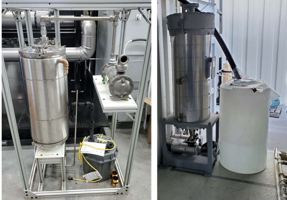
Figure F-2. Photographs of the water seal and condenser, which will be placed outside the shipping container (left) and the distilled water recycle tank (with appropriate insulation and line trace heating) inside the container for freeze protection.
