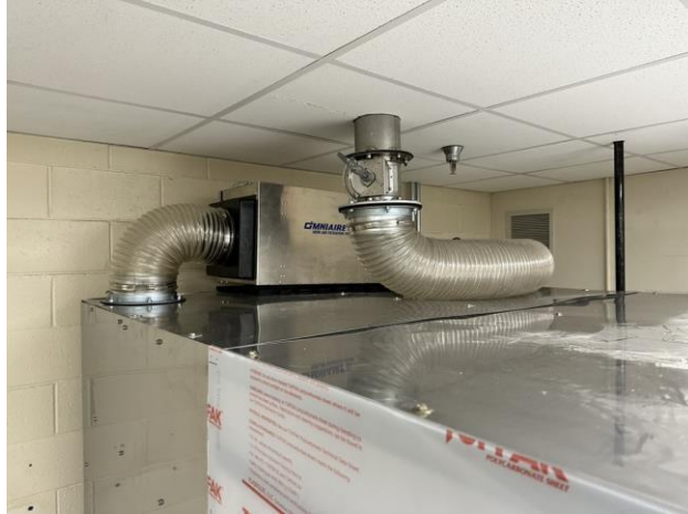
Installation complete of HEPA exhaust blower
