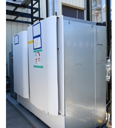
Bloom Energy 100\text{ kW}_{\text{eDC}} HTE Stack Module
