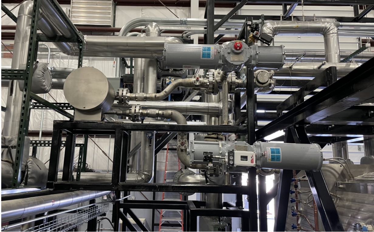
Figure 7. MAGNET-TEDS HX installation photo.
