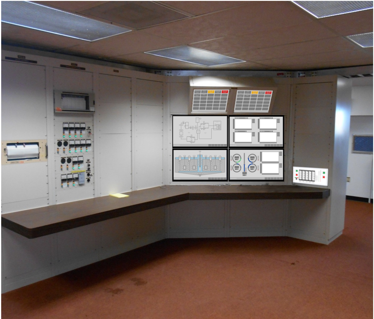
Figure 59. Graphic of control room with MARVEL screens and analog meters.
