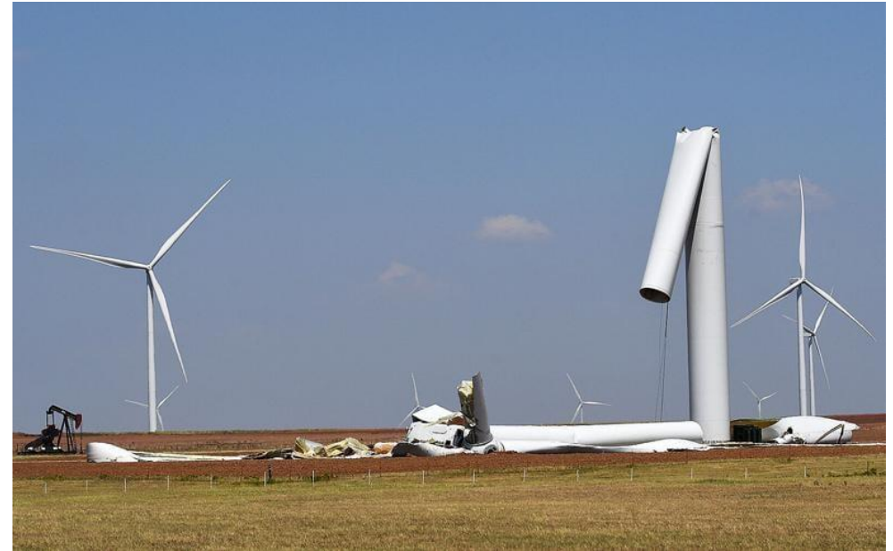
Critical failures can lead to severe physical damage.
